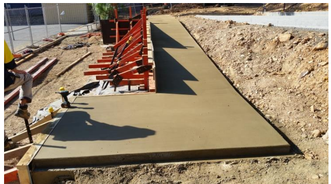
Construction of access way
