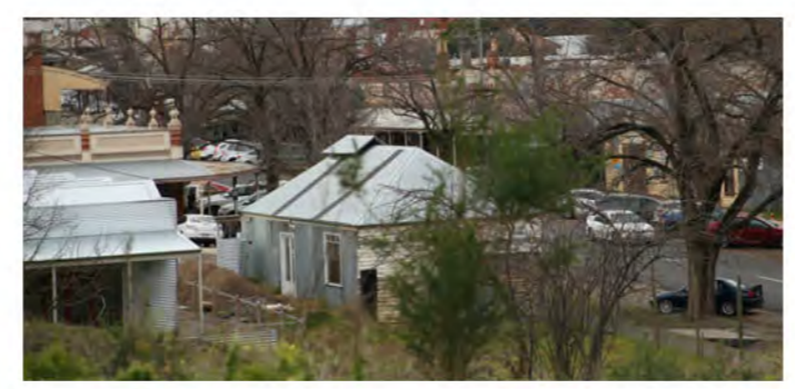
HIGH ST. X SPRING ST. NEW PROJECT AND ROOF RESTORATION
