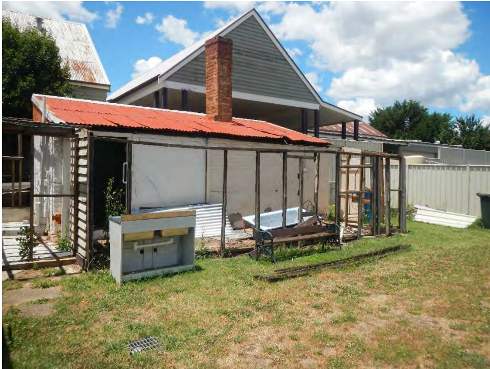
Rear section of existing dwelling to be removed
