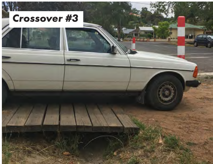
Timber crossovers are acceptable providing they meet the requirements of AS 1428.1 - 2009 Clause 7.2.
