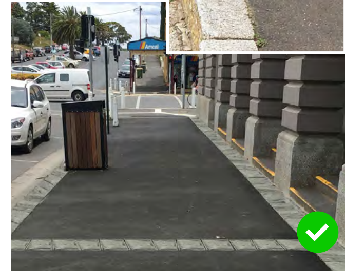
A small amount of banding across an asphalt footpath may be appropriate in feature locations, however bands should be used sparingly and made from local rough stone to match kerbs.
