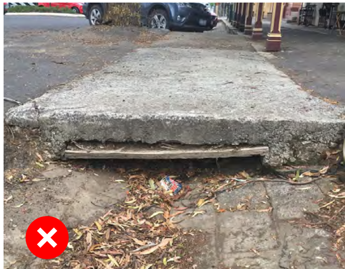
Crossovers in poor repair run the risk of blocking water flow and impacting drainage.
