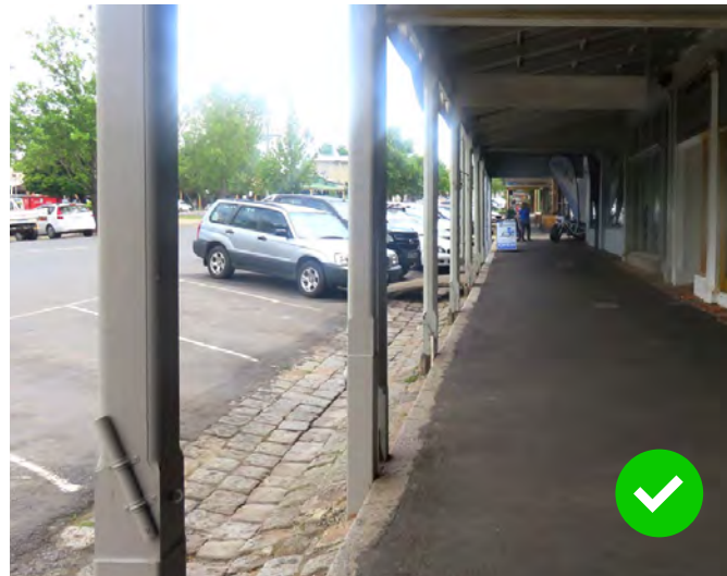
Asphalt paving is inexpensive, durable, easy to replace and does not draw attention away from the built form.
