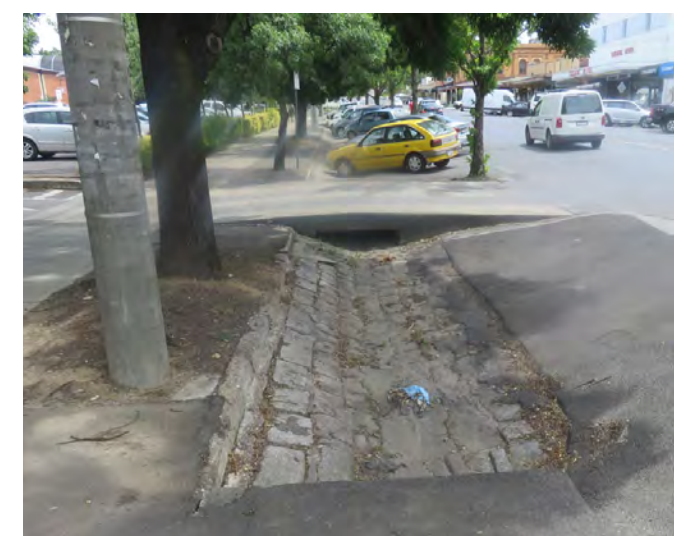
Hargraves Street at Forest Street: Stone channels set in wide, asphalt covered kerb extensions are prime candidates for water sensitive urban design approaches such as rain gardens.
