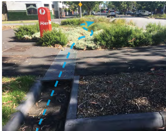
A rain garden where storm water is channeled into a planted kerb extension and allowed to permeate to a certain level before entering the storm drain system.
