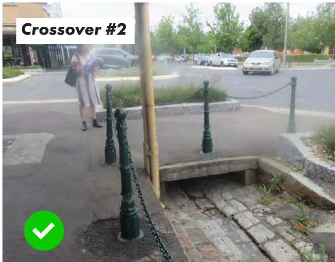
Asphalt on top of a rectangular culvert is acceptable.
