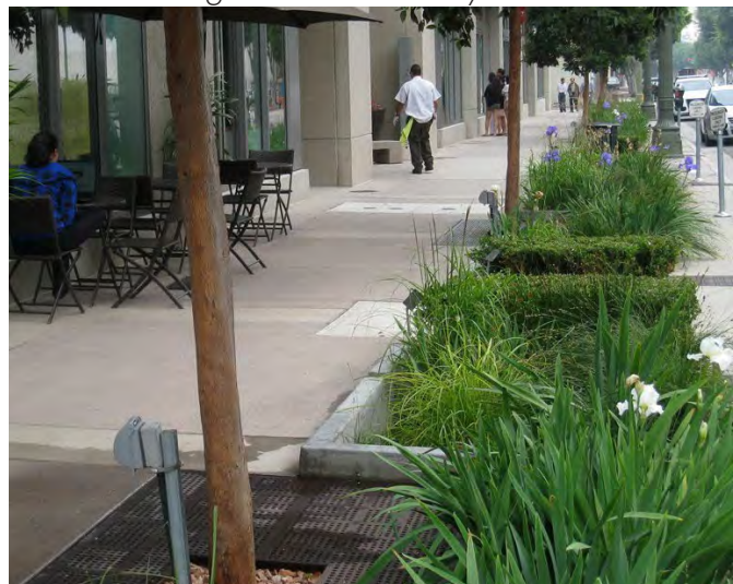
Rain gardens can fit within the cross-section of the footpath
