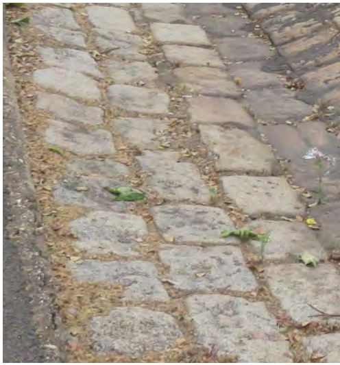
Footpath material #2: Stone banding used sparingly in the footpath and on pedestrian crossings to match local stone.
