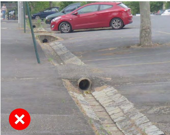
Make-shift asphalt crossovers compromising the stone channels are not acceptable. The crossover must be a stand alone component.
