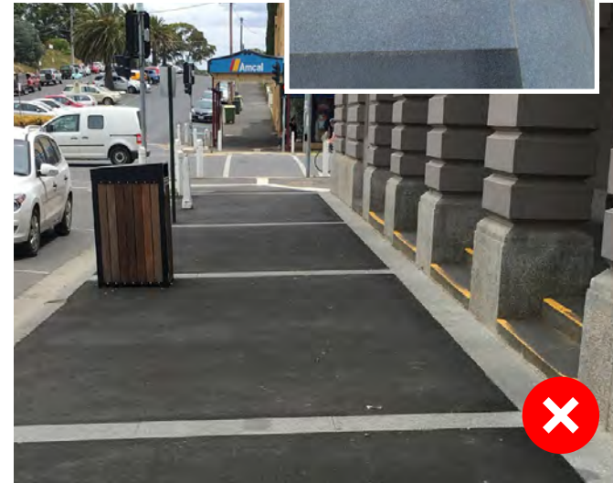
The sawn stone used in this footpath treatment does not match the existing stone in the town centre. While stone still needs to meet accessibility standards, the aesthetic should still match existing stone.
