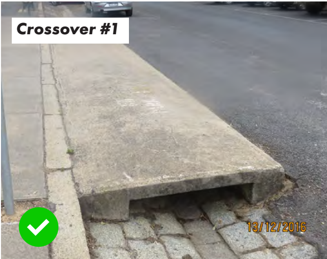
Concrete crossover with a rectangular culvert across the stone channel is acceptable.
