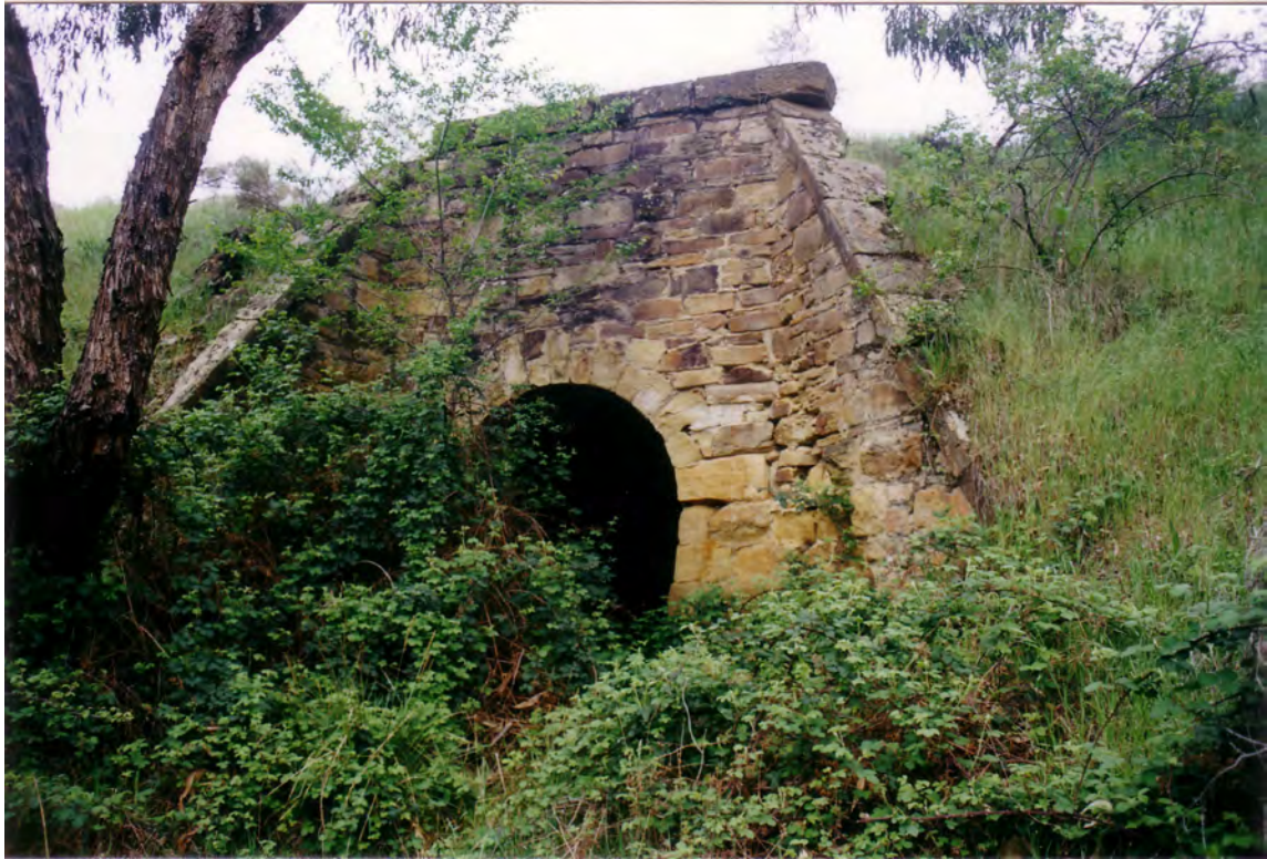
Stone Culvert, Vaughan Chewton Rd. Photograph Wendy Jacobs 1998
