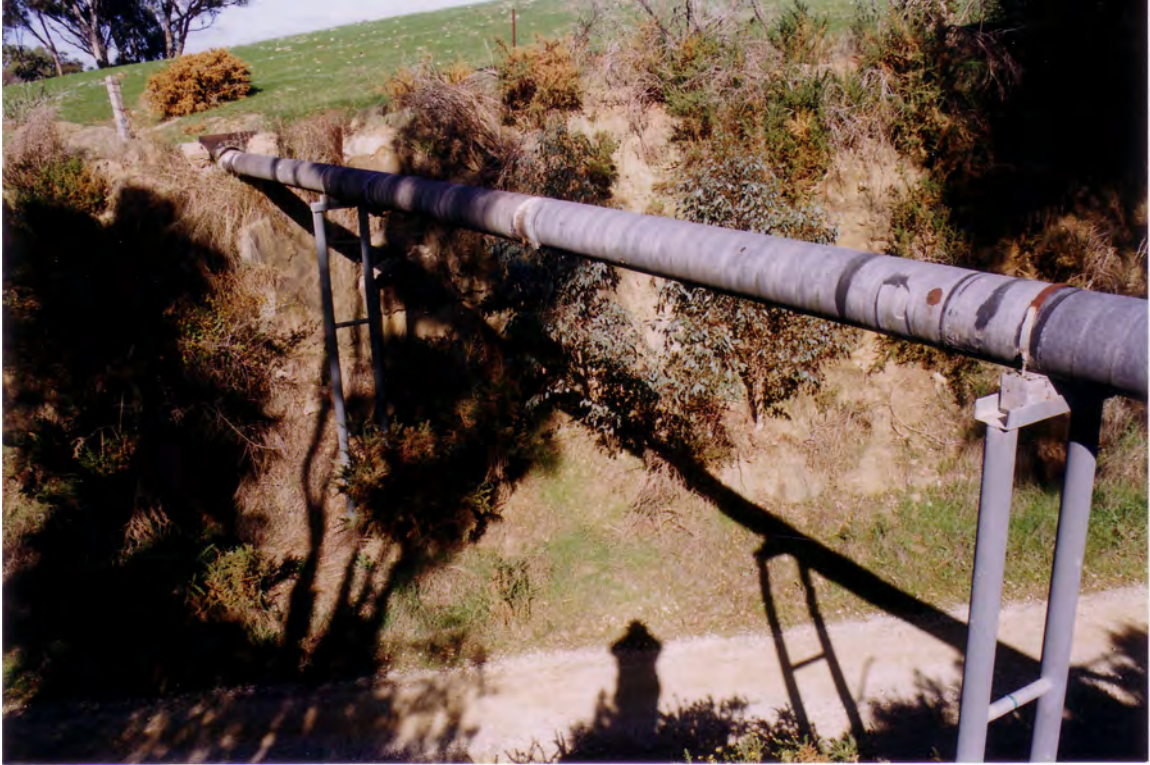
Flume over Fords Road, Campbells Creek Photograph Wendy Jacobs 1998
