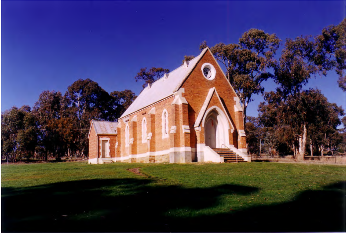
Sandon Catholic Church Photograph Wendy Jacobs 1998
