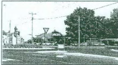
Fig 18: Prominent corner site: potential redevelopment site
