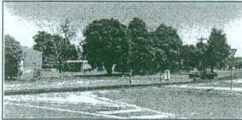
Fig 19: TXU depot: inappropriate use of town centre entry site
