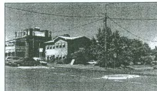
Fig 11: Potential Development site: Lyttleton Street
