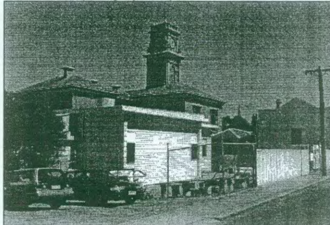
Fig 15: Relocation of obtrusive telecommunications building would enable creation of Post Office plaza.
