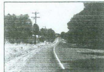
Fig 9: Duke Street - Eastern entrance
