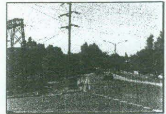
Fig 16: Johnstone Street - Power transmission sub station is visually obtrusive. Screen planting recommended.
