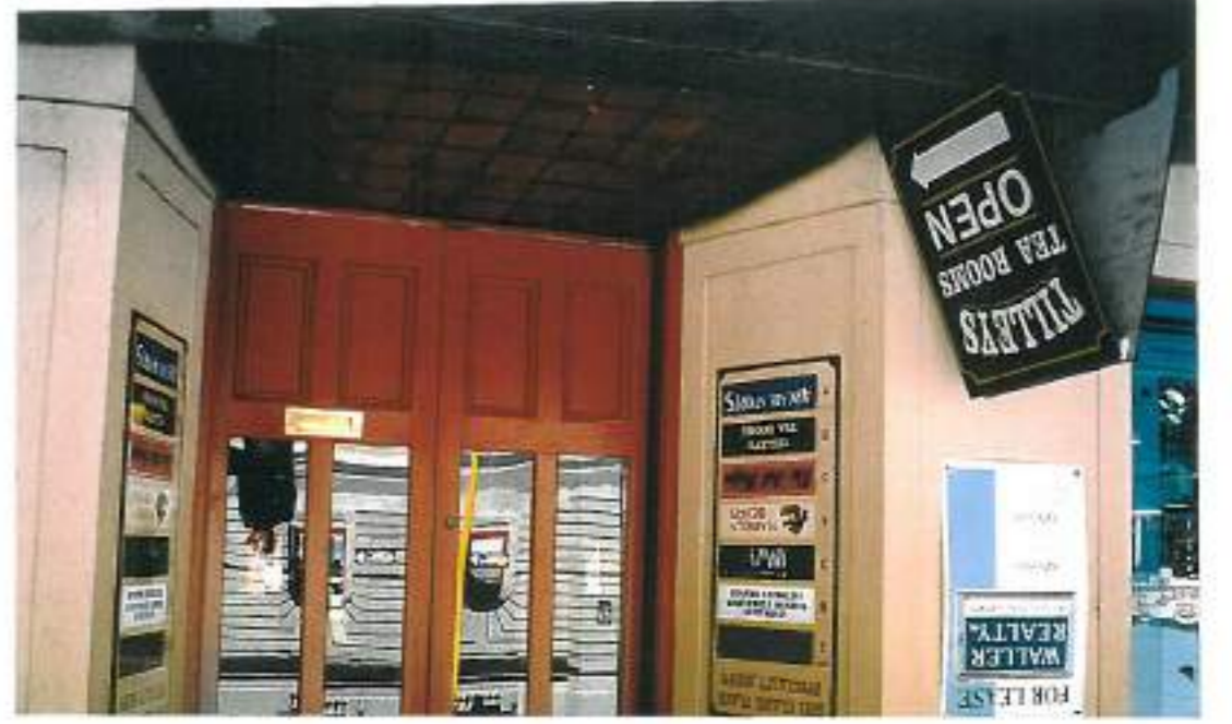
This entry has a problem with glass reflection which prevents passers by from seeing in.
