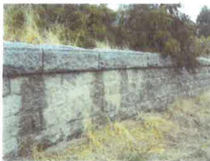
Historic granite retaining wall along Forest Creek
