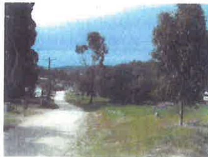
Unsealed side street
