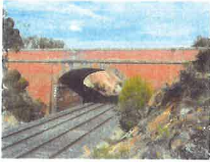
Historic brick railway bridge
