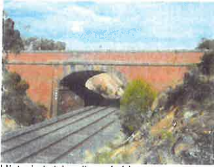
Historic brick railway bridge
