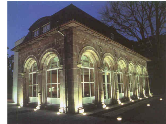
Figure 10 Example of Façade Lighting to Heritage Building
