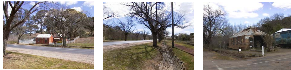
a. View northward along High street with stone gutters and elm trees b. Southwest view of first building along High St from the south, Mt Tarrangower in background c. Shed at prominent location in need of maintenance
