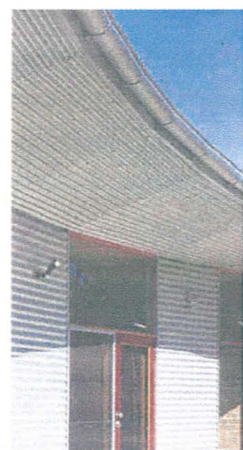
Figure 21. Contemporary use of corrugated iron
