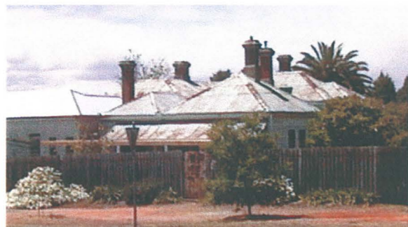
Figure 15. an example of the roofscape that commonly appears throughout Maldon's residential areas with verandah, pitched roof and chimneys.
