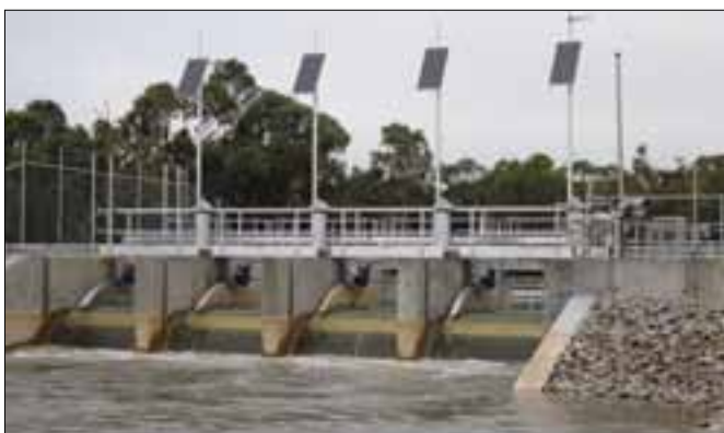
Hipwell Road Offtake regulator delivering environmental water into Gunbower Forest, June 2014
