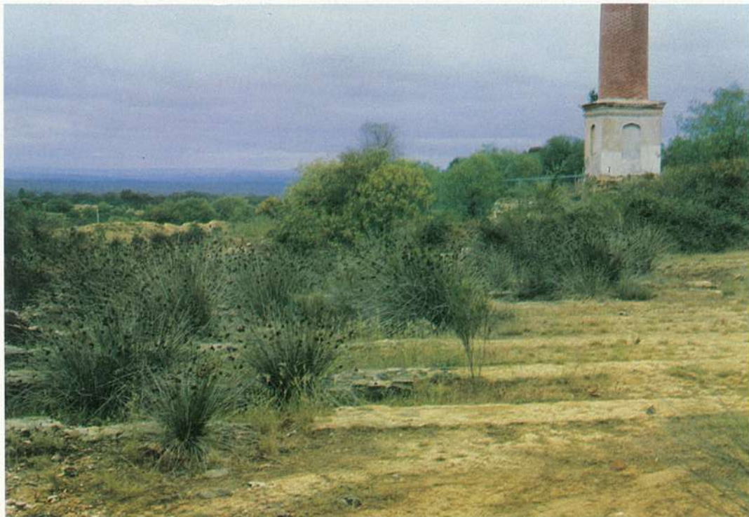
These foundations and chimney are all that remain of the once flourishing Beehive Mine. The stack is one of the largest surviving on any Victorian goldfield.
