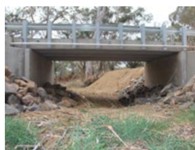
School Road Bridge
