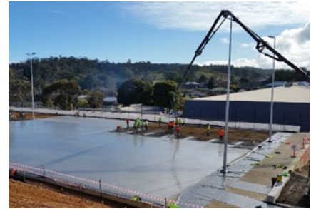
Construction well underway at Wesley Hill
