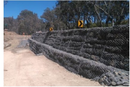
New gabion wall along Harcourt Sutton Grange Road
