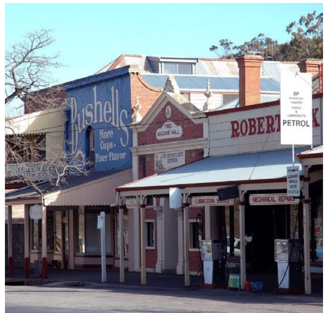
Work is set to continue on the Maldon Streetscape Project
