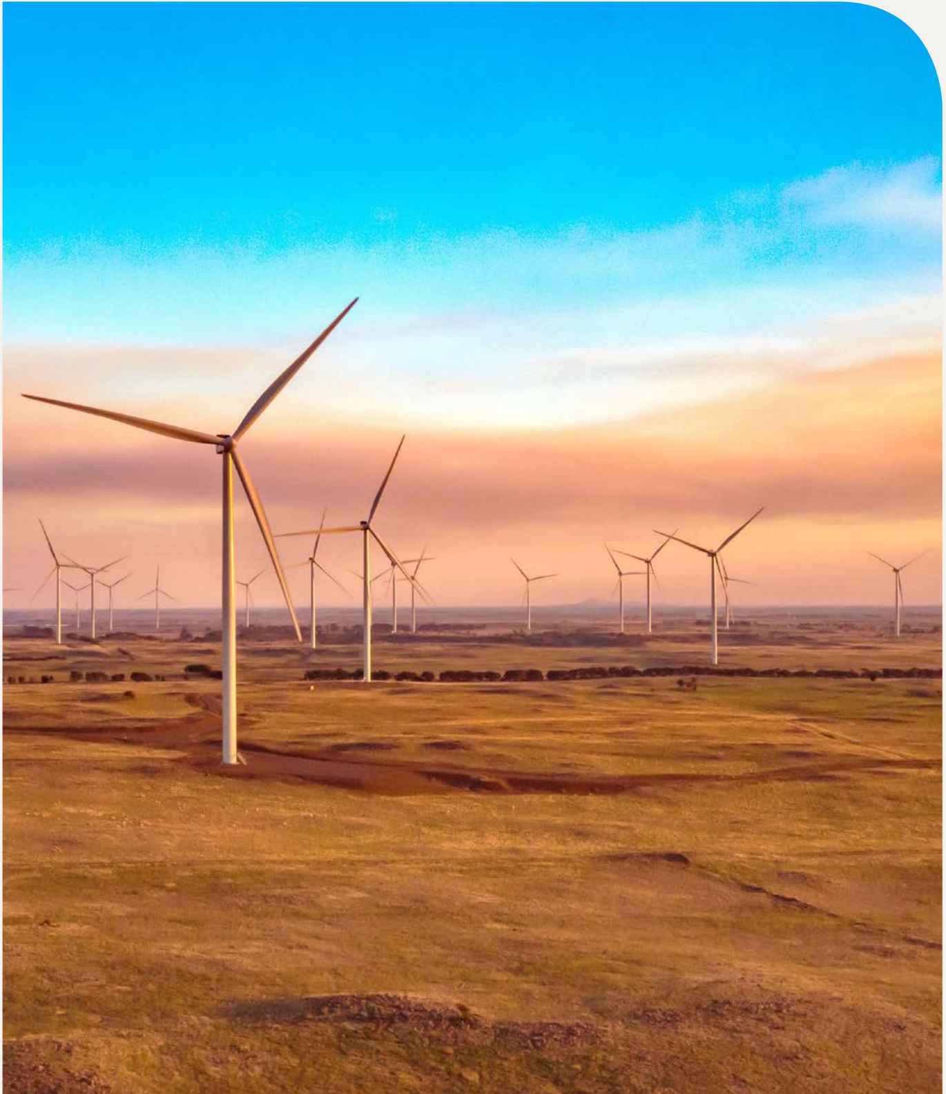
The Dundonnell wind farm near Mortlake.
