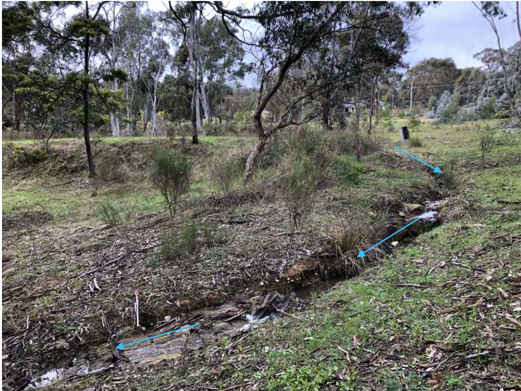
Photo 15 – View S along dam spillway channel
