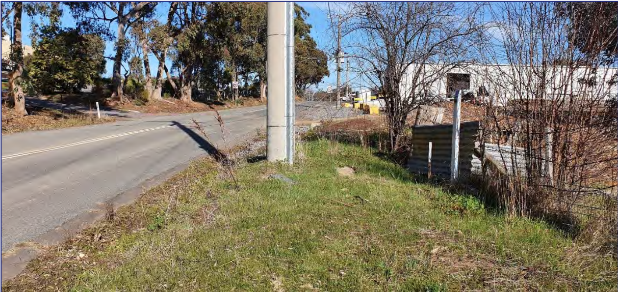
Figure 15: Sight Distance to the South of Main Carpark Crossover (145m, limited by the crest)
