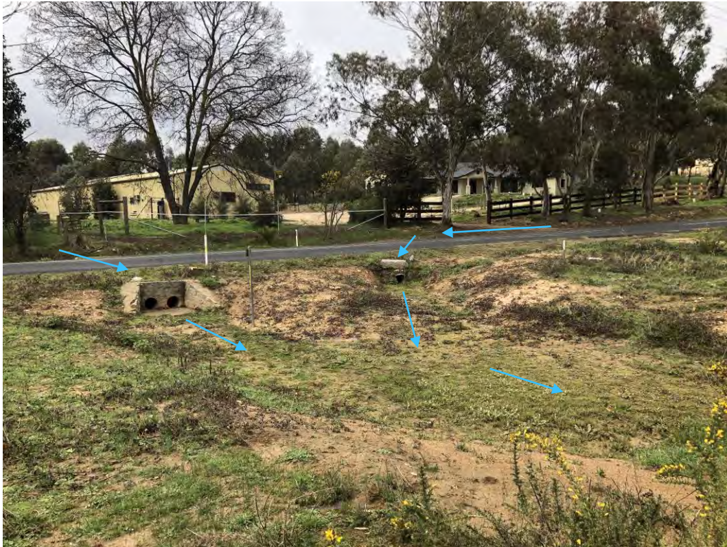
Photo 1 – View SE towards culverts under Blakeley Road
