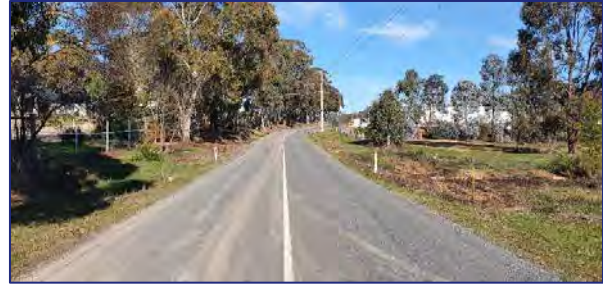
Figure 6: Blakeley Road – view south
