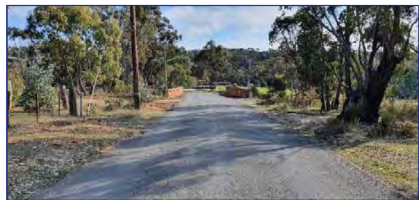
Figure 8: Sawmill Road – view west
