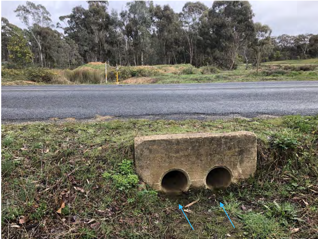
Photo 7 – View SE towards culverts under Blakeley Road
