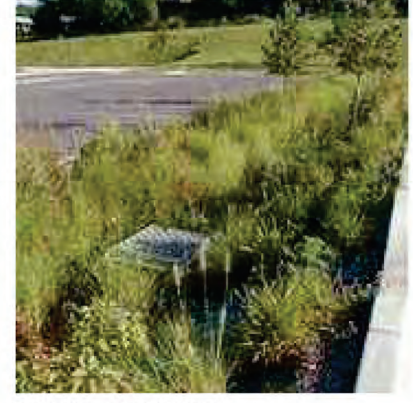
WSUD BIO-SWALE IN CAR PARK
