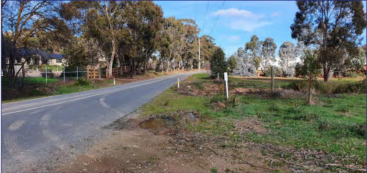
Figure 17: Sight Distance to the South from the location of the Secondary Carpark Crossover (Approx. 155m)
