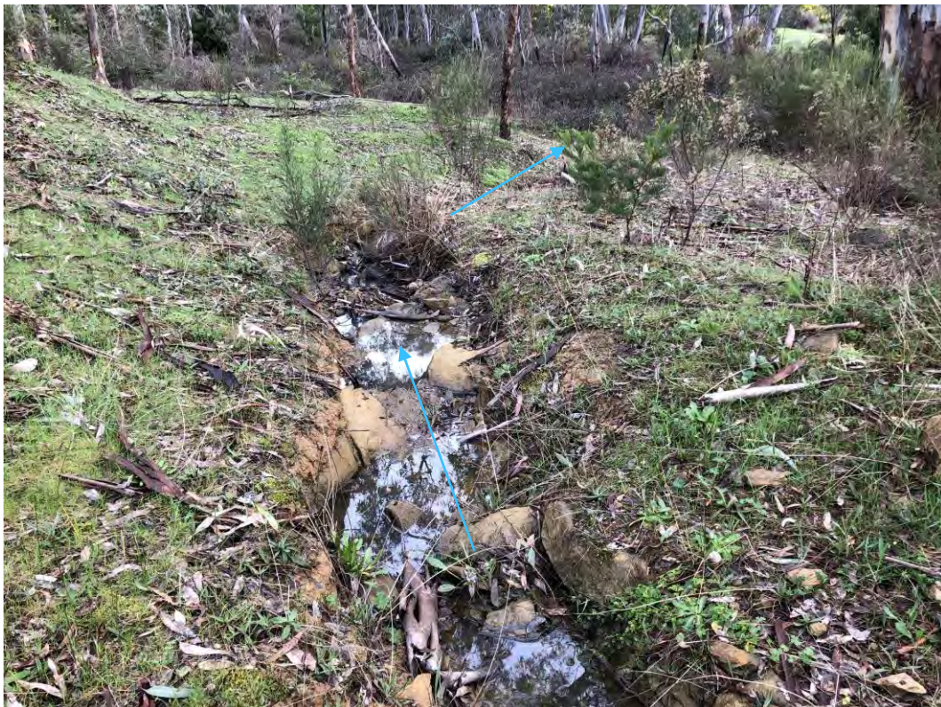
Photo 14 – View W along dam spillway channel
