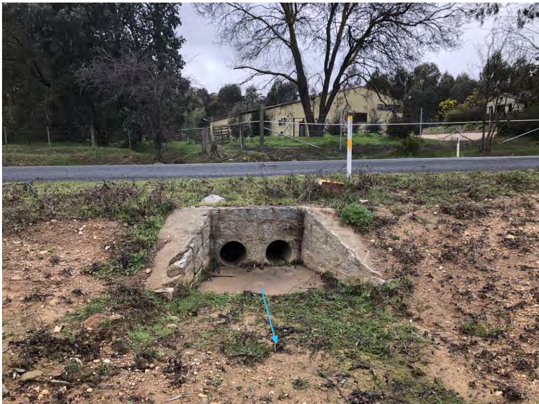
Photo 2 –Blakeley Road Culverts on Barkers Creek Tributary (twin ~375mm RCP)
