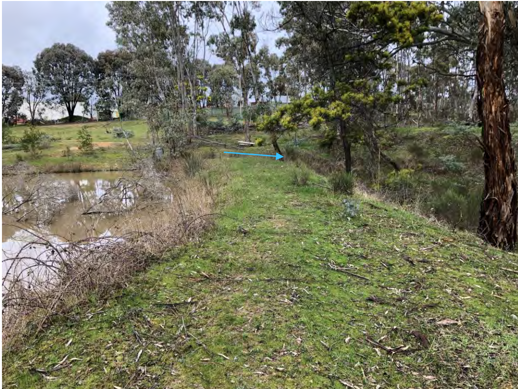
Photo 11 – View S along dam embankment
