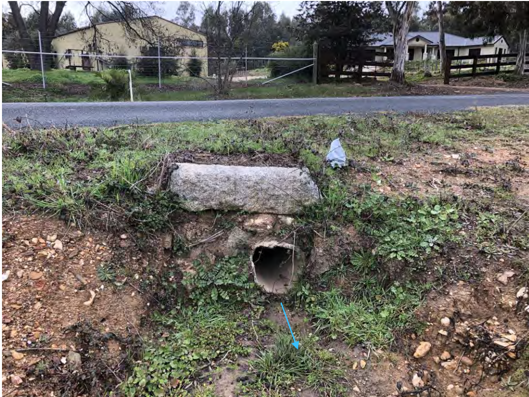
Photo 3 – Blakeley Road Culvert South (375mm RCP)
