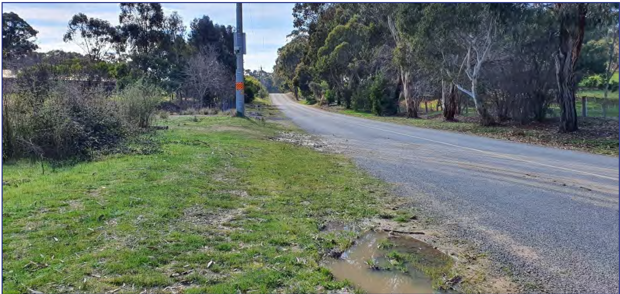
Figure 16: Sight Distance to the North of Overflow Carpark Crossover (Approx. 250m)
