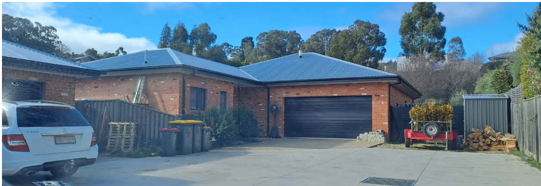
Figure 12. Site inspection photo taken by Callum Murphey
