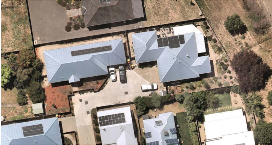
Figure 11. Aerial Evidence of Parking in the Common Property.
