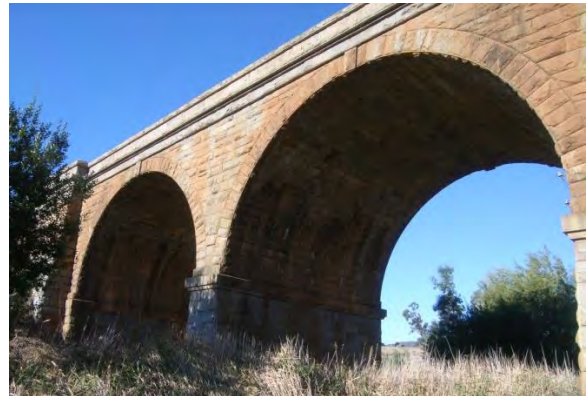
Figure 36: Bridge over Barkers Creek (2008)
