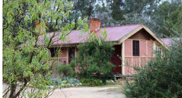
Figure 154: Powell's Prefabricated House, Campbells Creek (2014)
