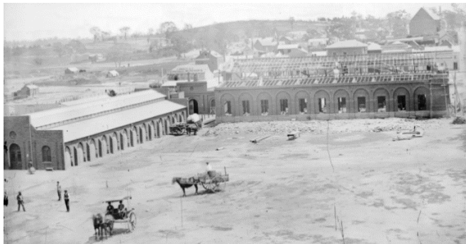
Figure 93: The three market buildings in Market Square, Castlemaine, 1861. The north market (right) is nearing completion. (Source: State Library of Victoria, accession no. H36596)
