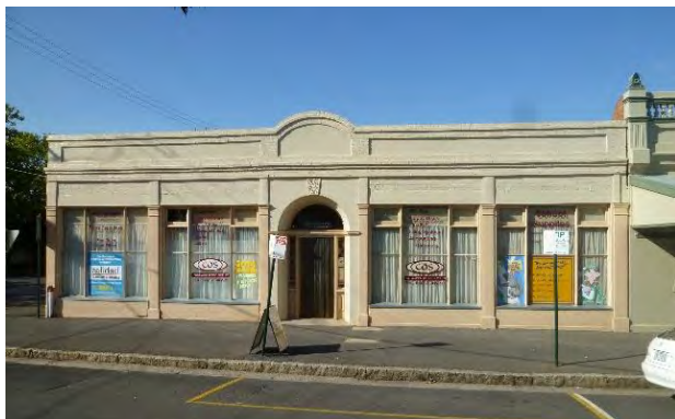
Figure 152: Former Midland Branch of the State Electricity Commission, Lyttleton Street Castlemaine (2014)
