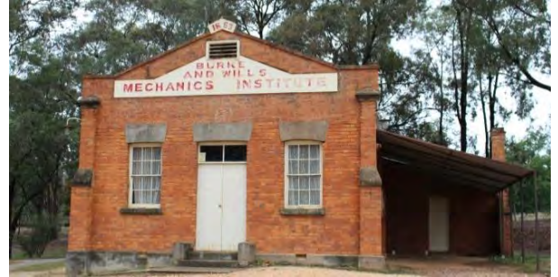
Figure 208: Fryerstown Mechanics' Institute (2014)
