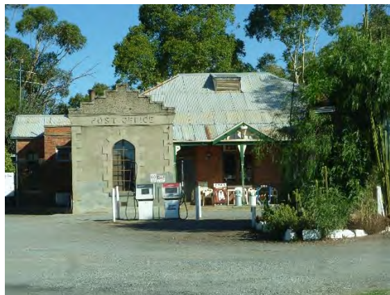
Figure 130: Former Post Office at Baringhup (2014)
