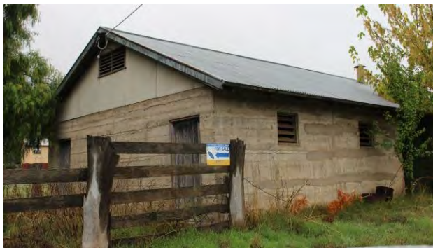
Figure 54: Concrete dairy in Parkins Reef Road, Maldon (2014)
