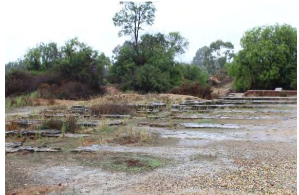
Figure 67: Foundations of the Beehive Mine at Maldon (2014)
