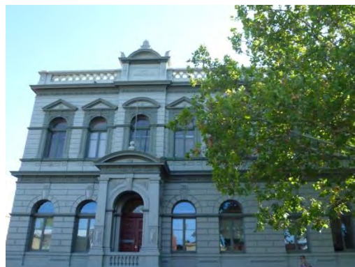
Figure 206: Former School of Mines, Castlemaine (2014)
