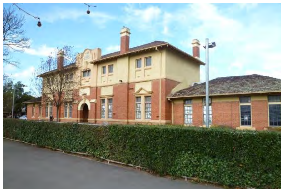
Figure 205: Former Castlemaine High School (2014)
