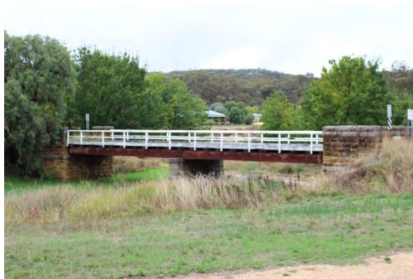
Figure 30: Zeal Bridge at Moonlight Flat (2014)
