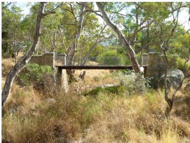
Figure 140: Granite bridge, Sutton Grange (2014)
