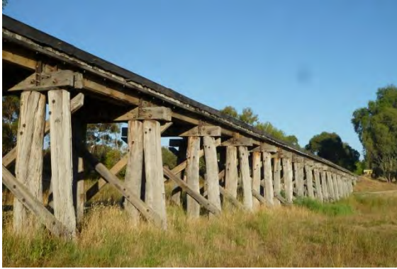
Figure 39: Timber railway trestle bridge over Campbells Creek Castlemaine (2014)
