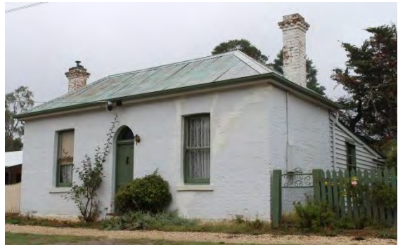
Figure 156: Early Victorian cottage at Chewton (2014)
