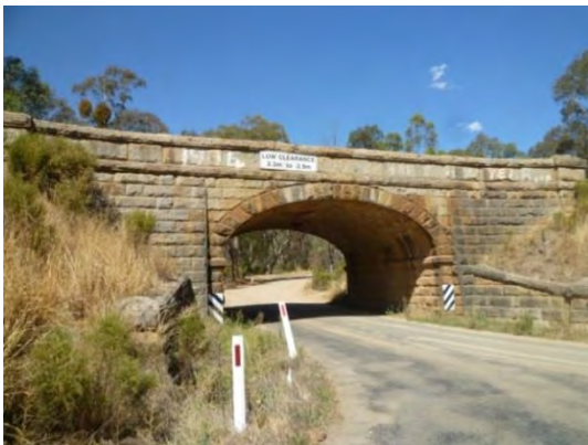
Figure 37: Specimen Gully Road Rail Bridge (2014)
