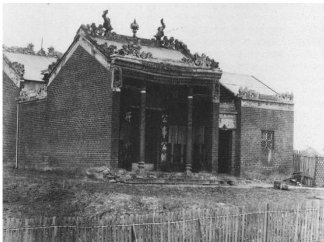
Figure 195: Joss house, one of several which stood near Forest Creek, Castlemaine (Source: Pioneers & Old Residents Association Collection in: G Hocking, Castlemaine from Camp to City , p143)
