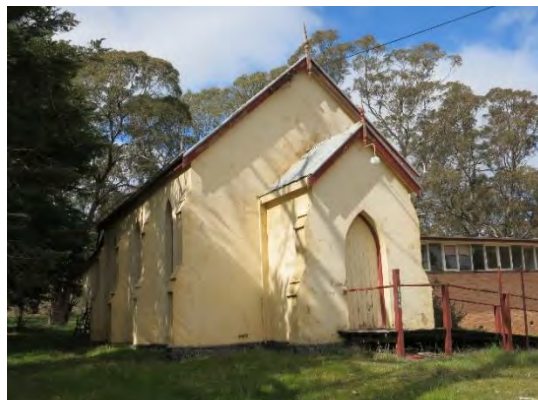
Figure 194: Former Harcourt Church of Christ, Midland Highway (2015)
