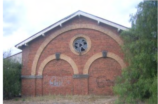
Figure 33: Castlemaine Station, goods shed (2008)
