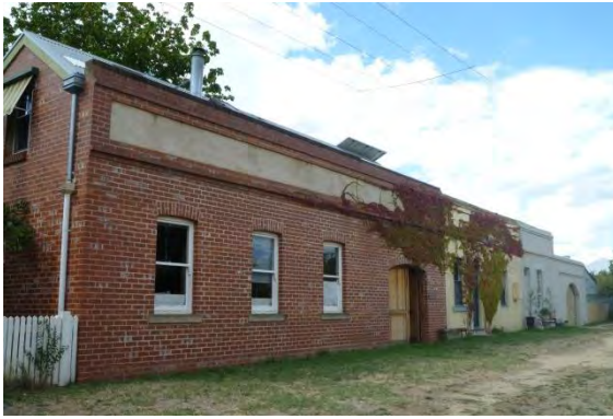
Figure 113: Former hotel, Fryers St, Guildford (2014)
