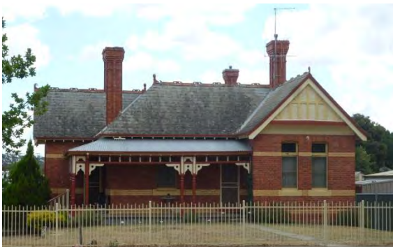
Figure 157: Federation period house at Newstead (2014)
