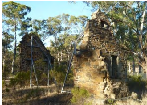
Figure 142: Stone ruins of the former Gower School (2014)
