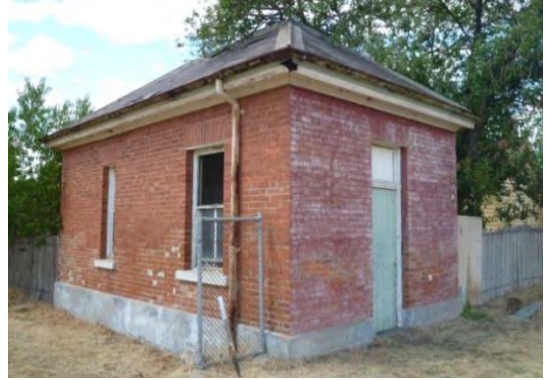
Figure 40: Newstead Station, former lamp room (2014)
