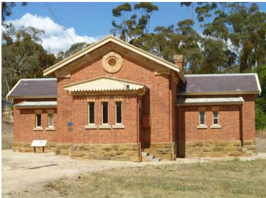
Figure 174: Former Newstead Courthouse, Canrobert Street (2014)
