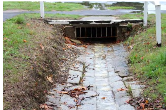
Figure 149: Urquhart Street, Castlemaine, culvert and stone drain (2014)
