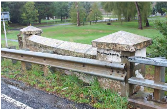
Figure 43: Bridge with rendered brick abutment High Street, Taradale (2014)
