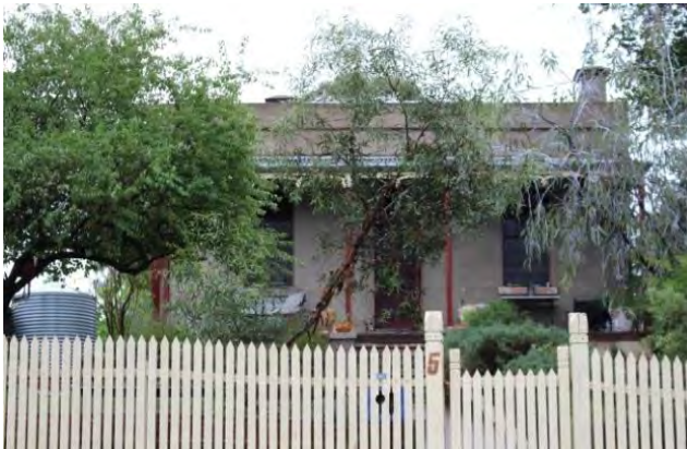
Figure 19: Former James Ah Coy house, Castlemaine (2014).
