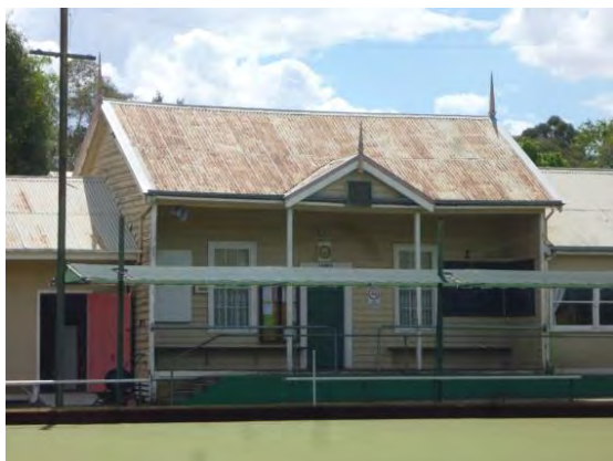
Figure 238: Patterson Pavilion at the Castlemaine Bowling Club (2014)
