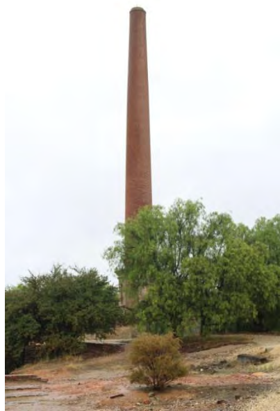
Figure 72: Chimney stack, 1861, of the Beehive Co. Mine at Maldon (2014)
