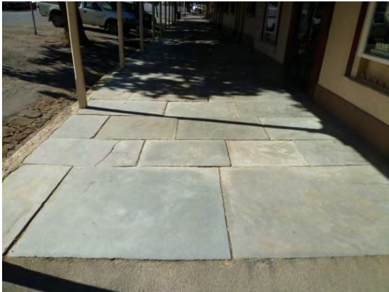
Figure 150: High Street, Maldon, early flag paving (2014)
