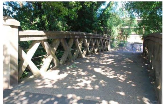
Figure 44: Concrete Truss Bridge, Castlemaine (Source: Victorian Heritage Database)
