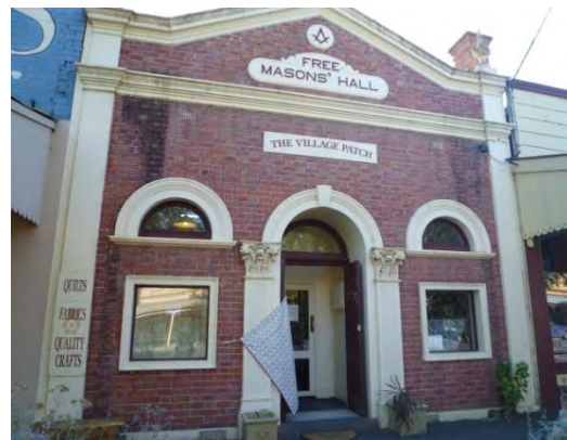
Figure 214: Former Freemasons' Hall, Maldon (2014)
