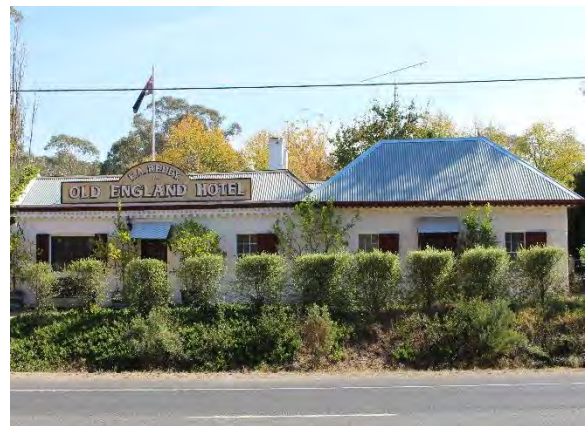
Figure 102: Old England Hotel, Barkers Creek (2014)
