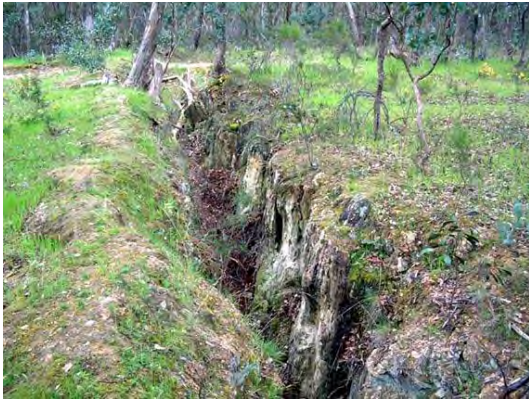
Figure 79: Channel cut through rock to supply water to gold workings (Source: Coliban Water website)
