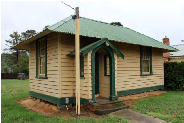
Figure 27: Former toll house at Campbells Creek (2014)
