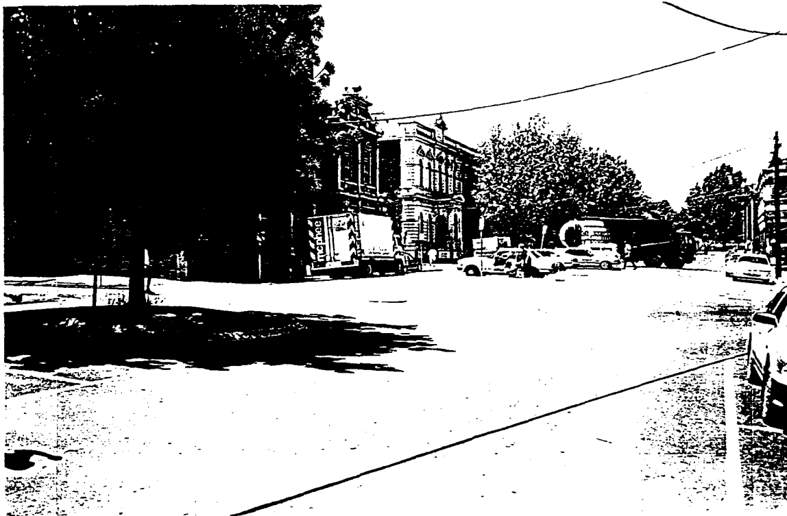
Lyttleton Street at Frederick Street
