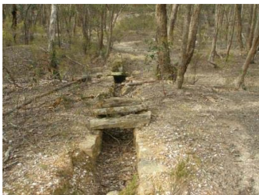
Figure 25: Remains of the stone flue at the Tubal Cain mine site in Sailors Gully.
