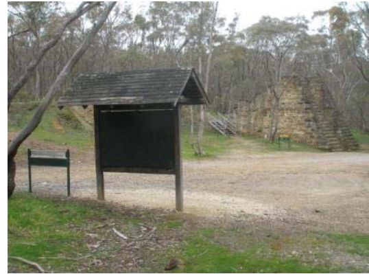
Figure 8: View of Garfield Wheel foundation and back of information shelter.
