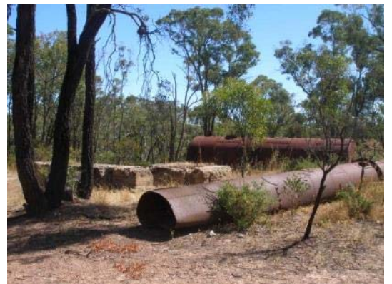
Figure 19: Remains of boiler, siphon and concrete foundations at Wattle Gully Extension Mine.
