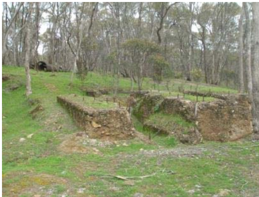
Figure 9: Engine foundation for winding gear on the Garfield trail.
