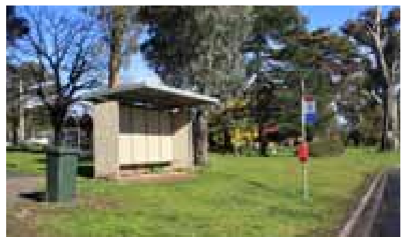
Existing bus stop on the Old Calder Highway
