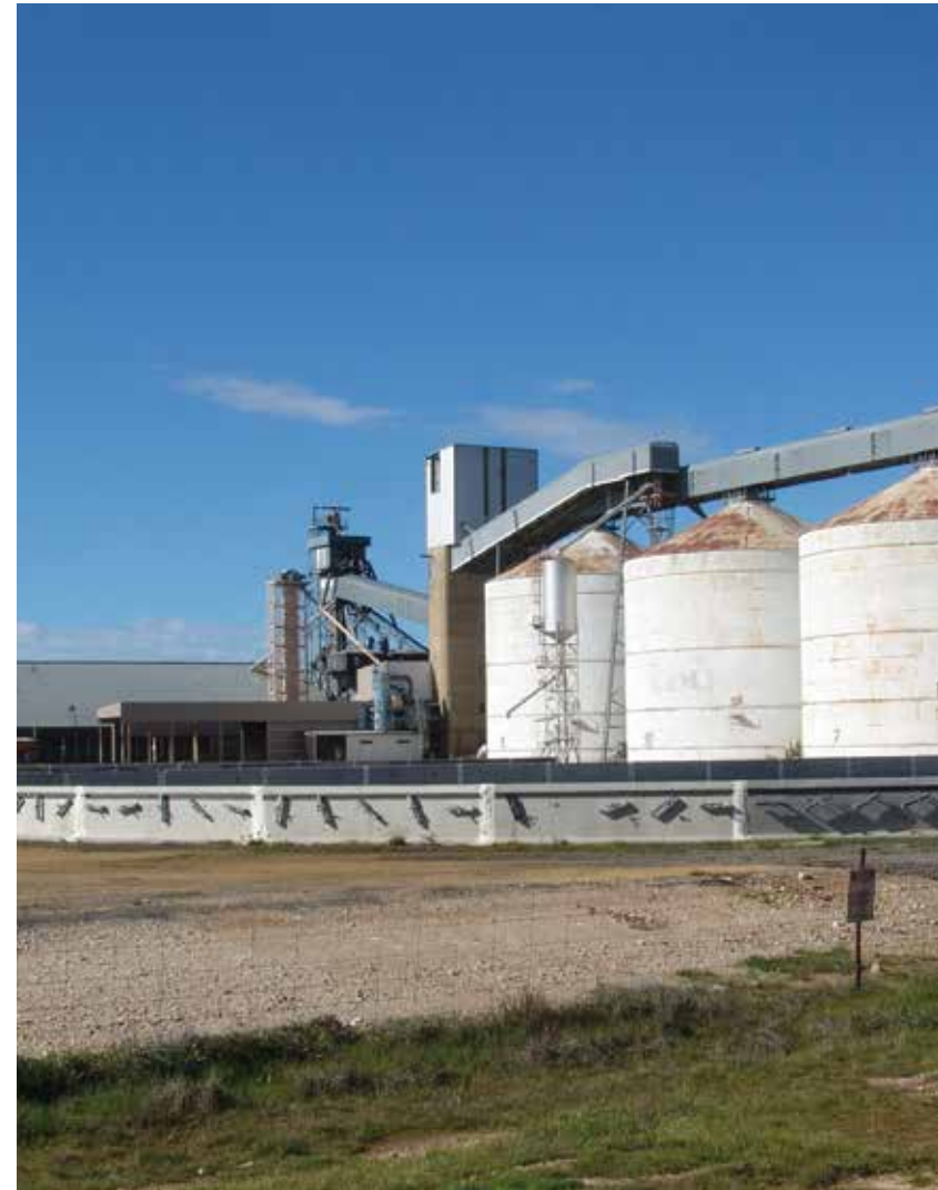
Dunolly Grain Handling Facility, Central Goldfields Shire
