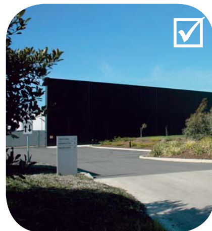
Figure 25: Visitor car parking is provided at the front, with other parking away from public view
