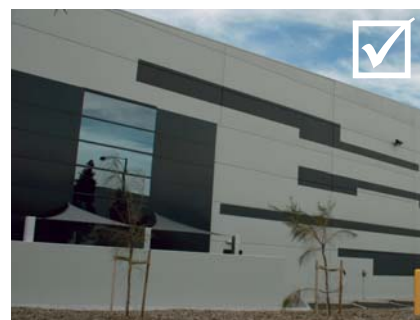
Figure 12: Blank tilt concrete walls articulated with pattern and colours provide visual interest
