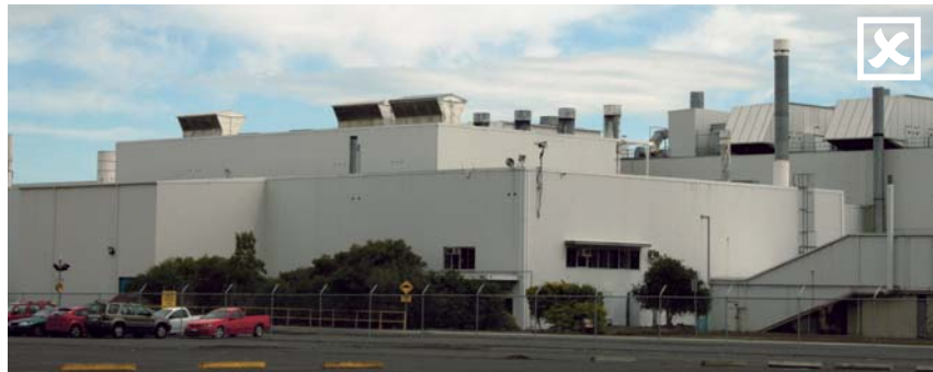
Figure 15: Ancillary fixtures should not be visible from public spaces and contribute to visual clutter
