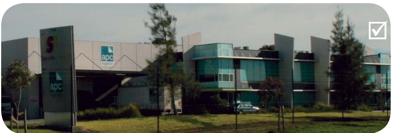
Figure 19: Muted colours present a good street address and ties different parts of the building together well.
