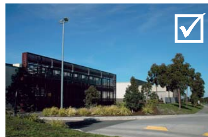
Figure 10: Interesting architectural detail provides good street address while also screening off excess solar heat gain
