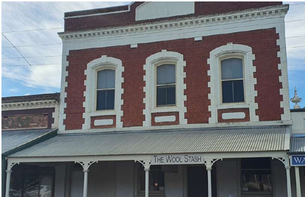
Figure 10. Note the replacement verandah with simple timber posts and timber fretwork that is based on the design of the original verandah. (Source: GML 2021)
