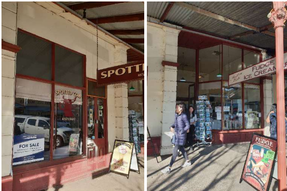
Figure 6. Views of 24 (left) and 22 (right) High Street, showing the replacement shopfronts. (Source: GML 2021)
