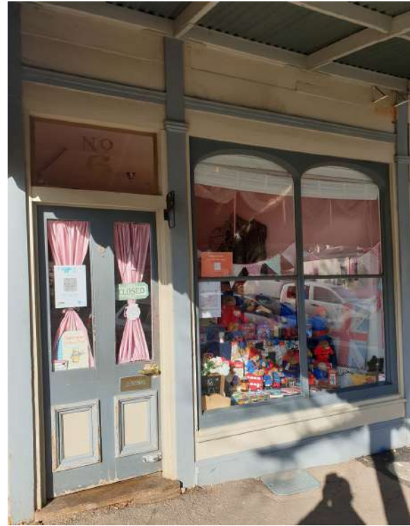
Figure 12. The ground-level façade retains decorative timber pilasters and cornices, original shopfront window and half glazed door with highlight. (Source: GML 2021)
