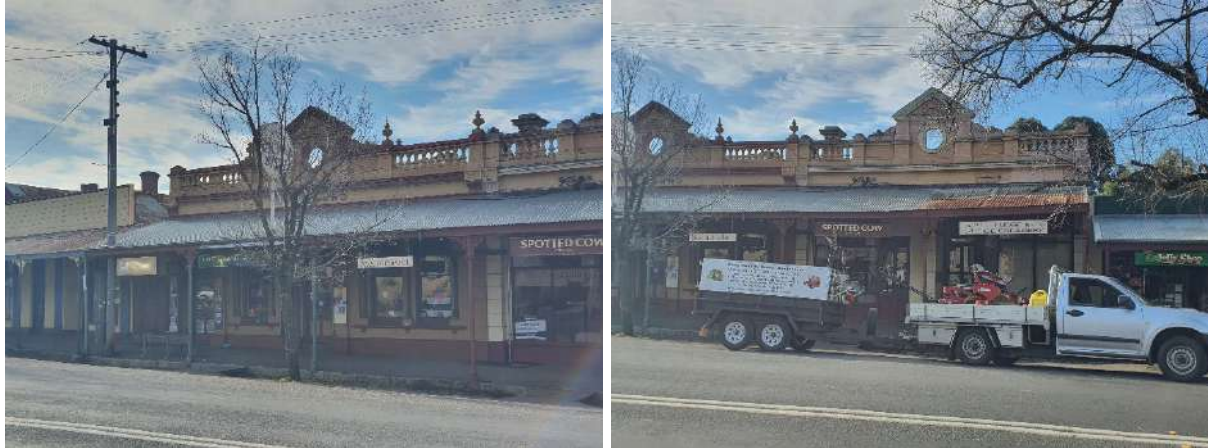
Figure 5. View of 26 High Street (left) and 22–24 High Street (right), Maldon. (Source: GML 2021)
