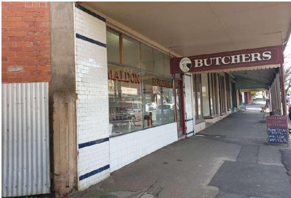
Figure 6. Note the aluminium framed shopfront likely dating from the early 1960s. (Source: GML 2021)
