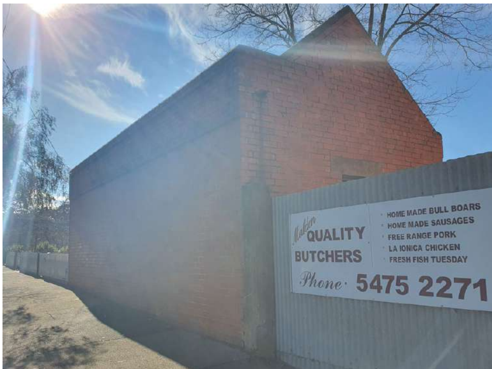
Figure 7. Former stables building in High Street. Note the clinker brick surrounds along the parapet on the street frontage. (Source: GML 2021)
