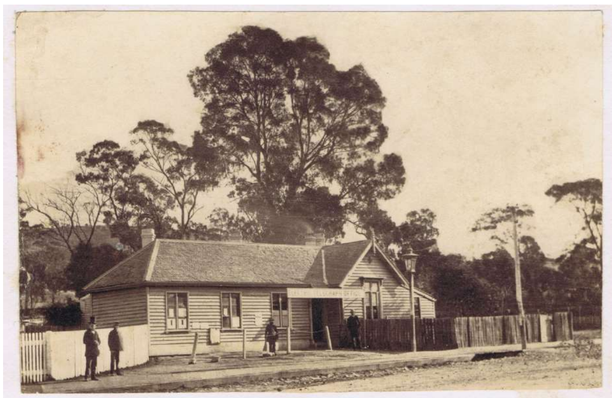
Figure 3. A closer view of the former post and telegraph building, c1869. (Source: MM&AA VMLD 4535)
