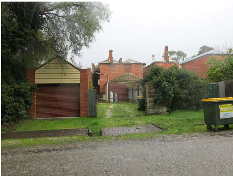
Figure 8. Rear of 22–26 High Street, note the timber section at the rear of 22 and 24 High Street. (Source: GML 2021)
