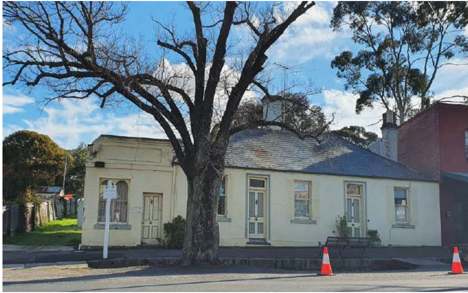
Figure 7. View of 61–65 High Street, showing the original 1857 section and 1877 addition to south. (Source: GML 2021)
