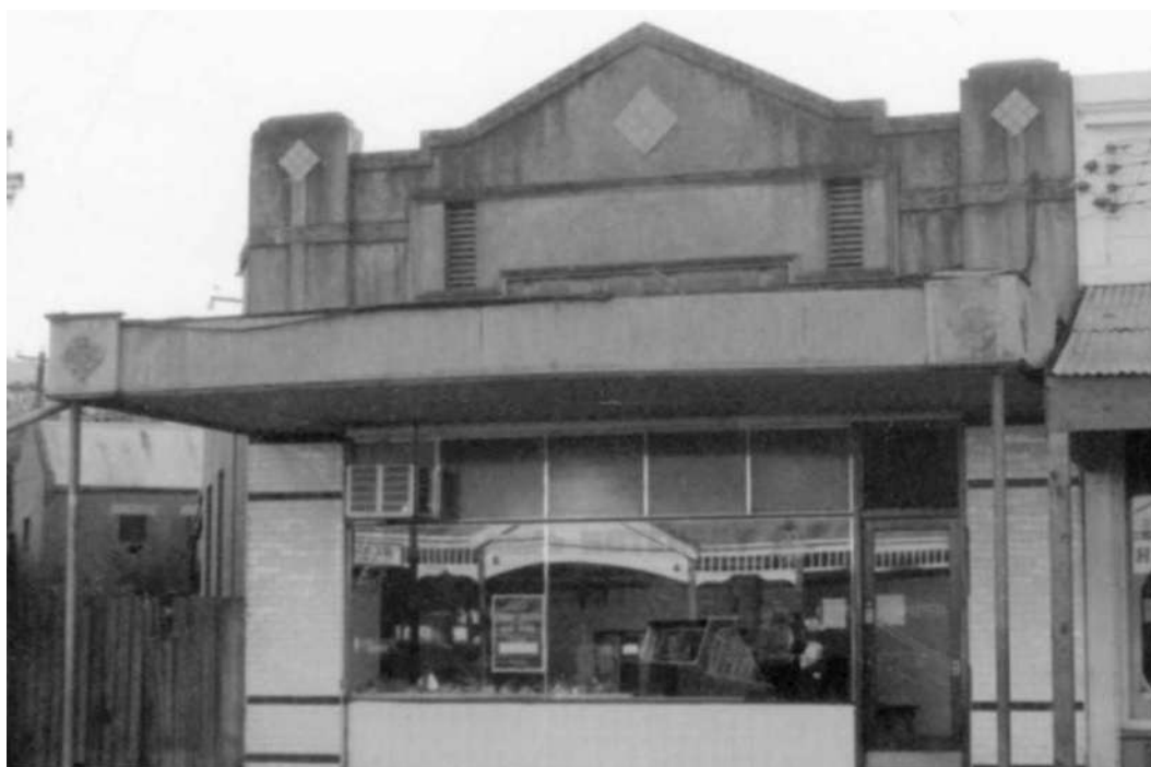
Figure 4. The subject building c1977, by which time the cantilevered verandah had been propped up with a metal pole at each end and the doorway moved from the centre to the side. (Source: Maldon Tours)
