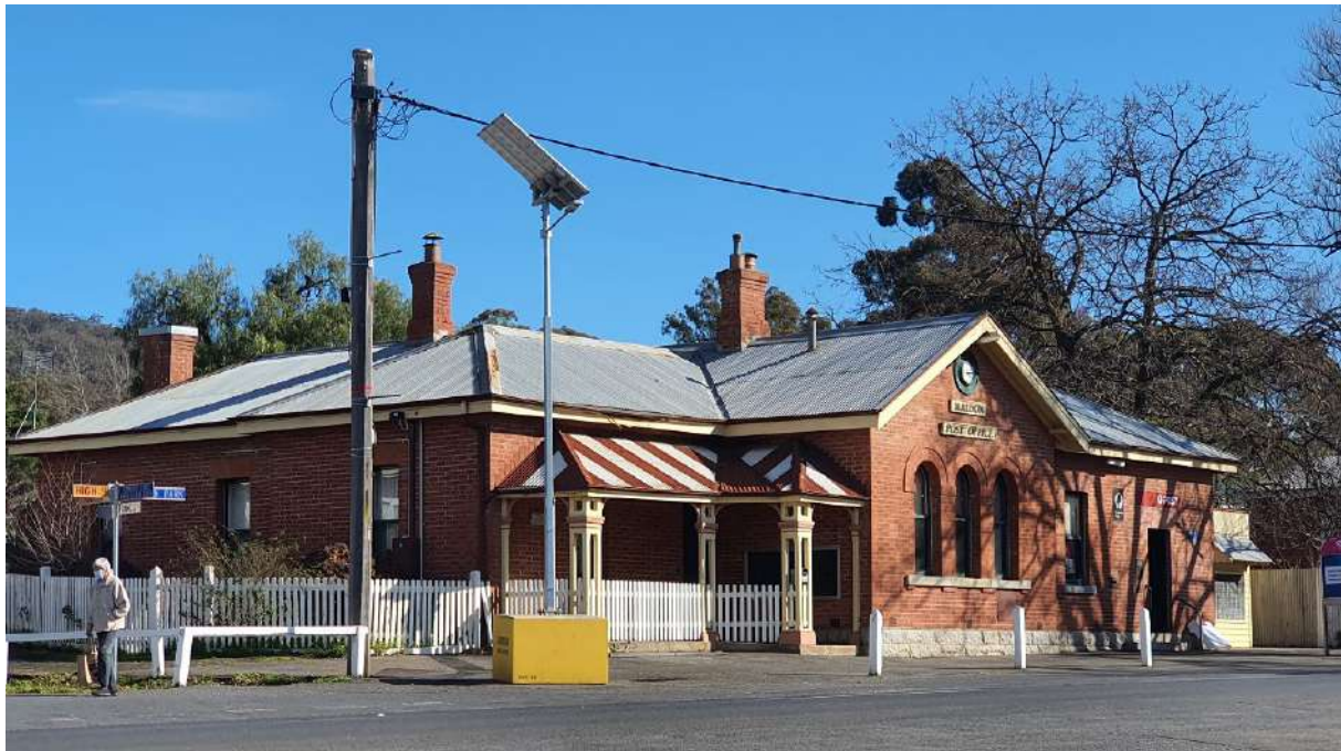
Figure 11. View from High Street, showing the projecting wing with the triple arched window, the signage and the clock, and the restored verandah. (Source: GML 2021)
