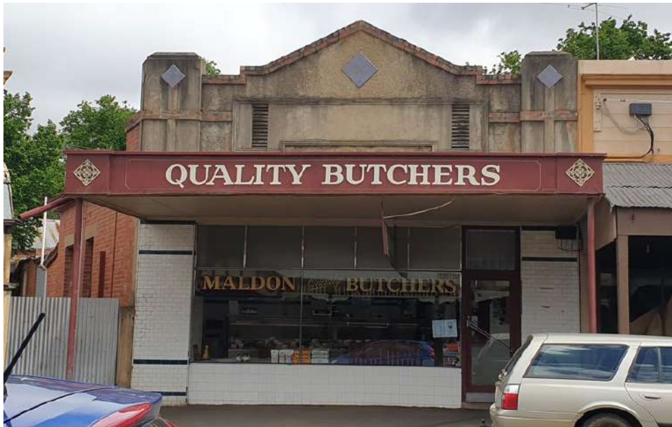
Figure 5. View of the 1927–28 shop from Main Street. Note the original parapet and west elevation. The verandah appears to be the early 1960s addition. (Source: GML 2021)
