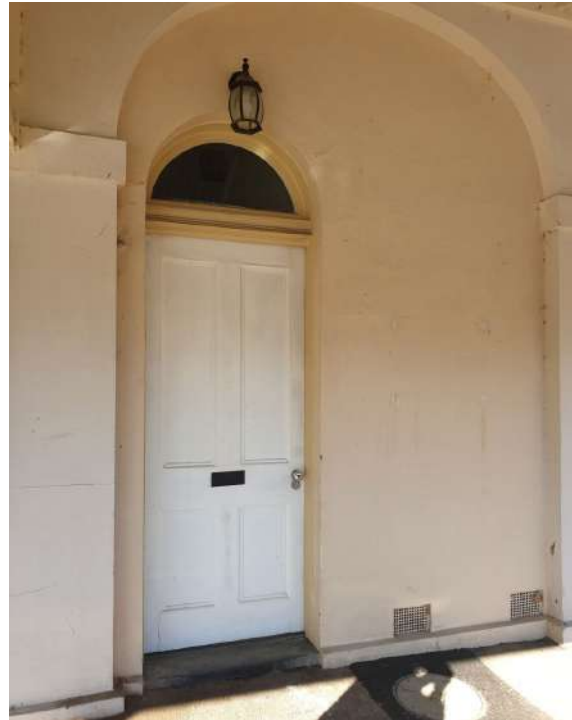
Figure 9. Original carriageway converted to a doorway in 1888. (Source: GML 2021)
