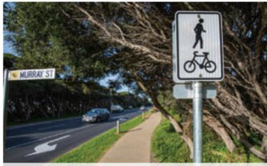
An aggregate pathway like this one provides a solid, durable, surface and is more sympathetic to heritage than concrete or asphalt shared pathway, Mornington Peninsula VIC
