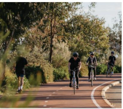
Bi-directional coated asphalt shared path. The red coating is more fitting with a heritage aesthetic than traditional uncoated asphalt - riverfront bike path, Perth WA
