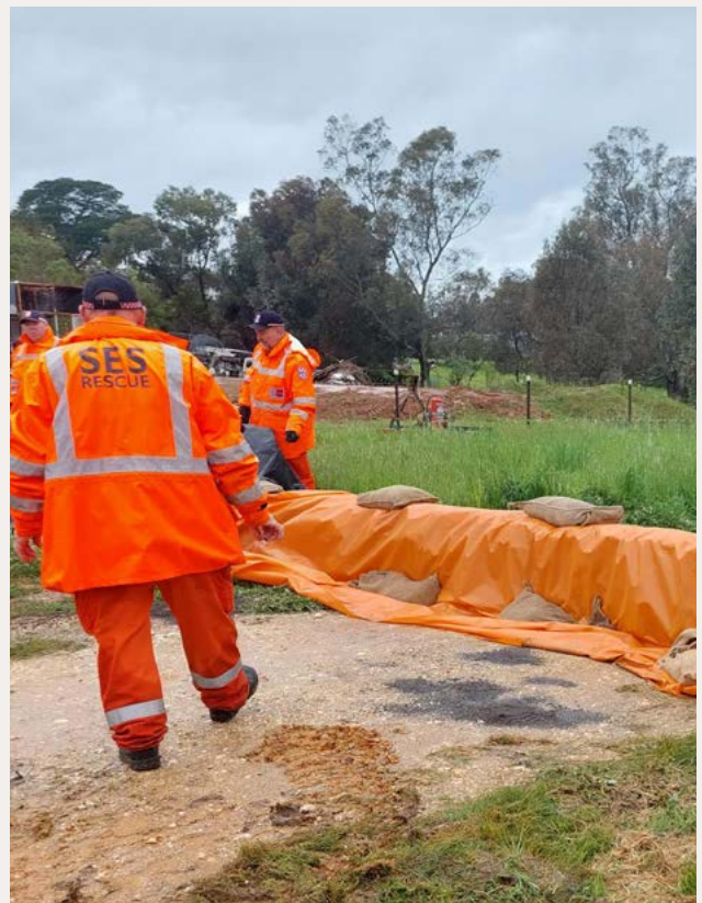
Sandbags being placed to prevent flooding.
