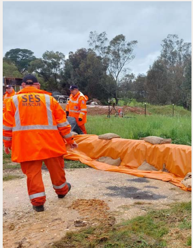
Sandbags being placed to prevent flooding.
